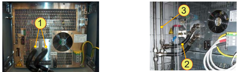
Fig. 46 Examples for liquid cooling using cooling liquid: 90 ° quick-release isolating valves -1- on a 32 kW power supply Hosing -2- and pipework -3- on a 32 kW power supply in a device cabinet.
